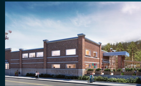
Community Center / Vacant Pharmacy
