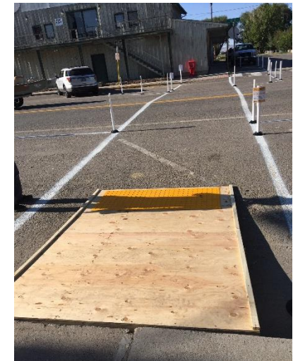
Temporary curb ramps
