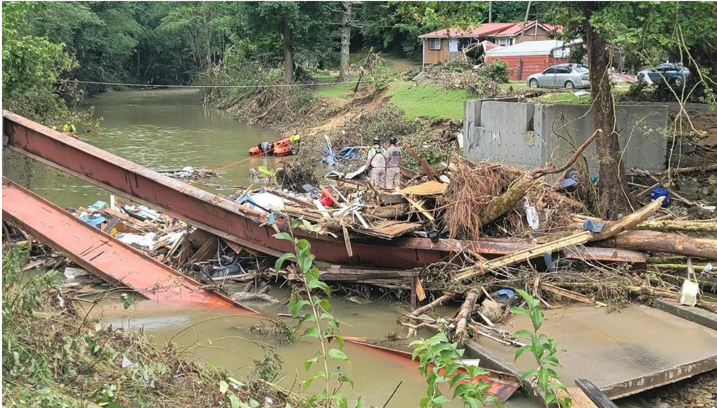
Flood damage and search operations near the Perry-Knott county area following the July 2022 Eastern Kentucky floods. Photo: LEX 18.
