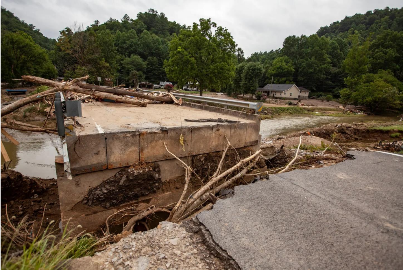
A bridge across Grapevine Creek at Chavies School Road in Perry County, Kentucky, heavily damaged by flooding on July 28, 2022. Photo by Ryan C. Hermens, Lexington Herald-Leader.
