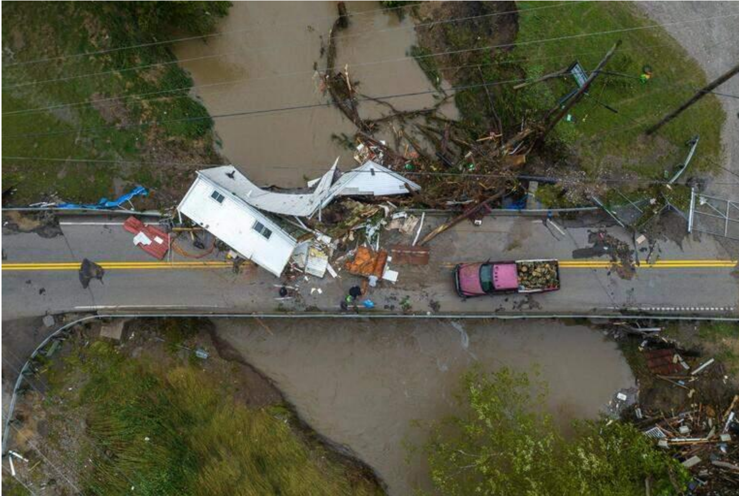
A house carried onto the KY 931 bridge over Sandlick Creek near Whitesburg, Kentucky, following the July 2022 flood. Photo by Ryan C. Hermens, Lexington Herald-Leader.
