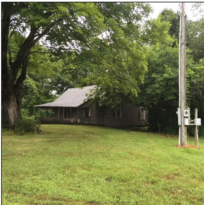
Figure 37. Many homes in Pope County are constructed with combustible wood components and although defensible space is generally good throughout the county, some homes are located immediately adjacent to woodland with overhanging vegetation.
