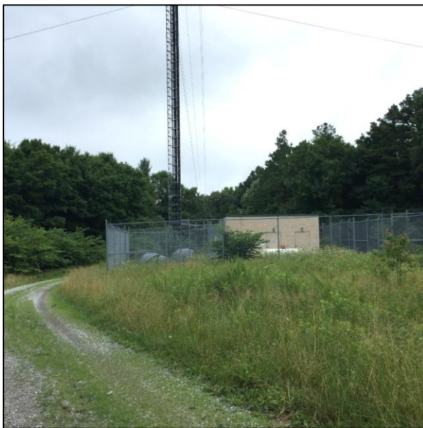
Figure 81. Communication site on Williams Hill.
