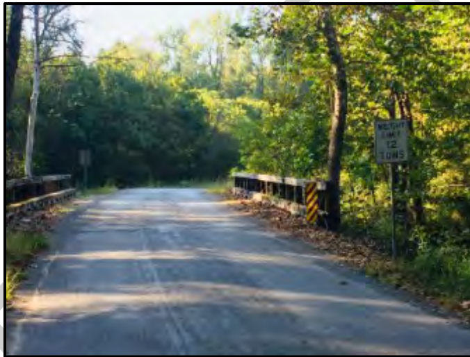
Figure 3.15. Bridge close to the Iron Furnace with weight limit.
