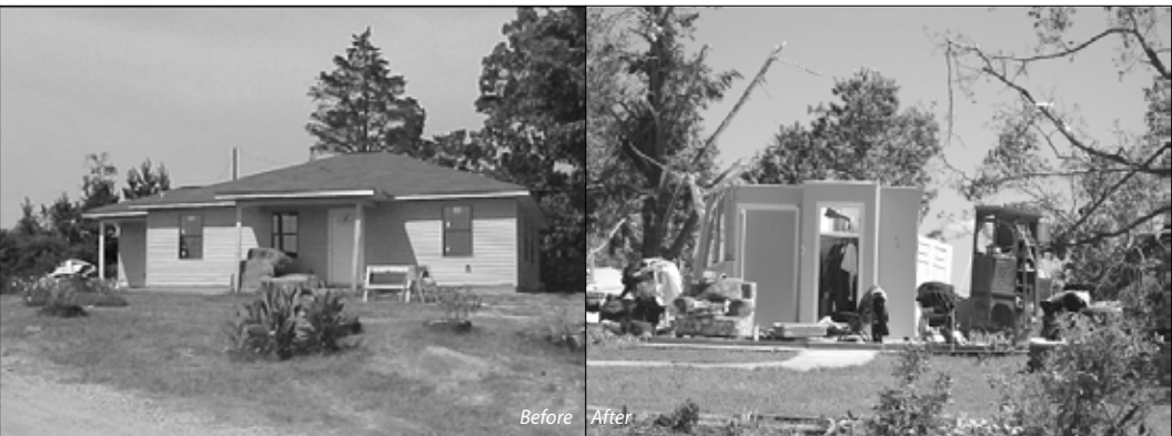
This home in Choctaw County, MS suffered damage during the tornado. Photos courtesy of GTPDD.
