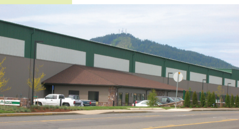
The new Murphy Plywood facility, re-opened in 2005.
