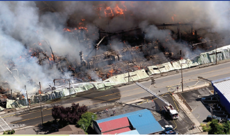
The 2005 fire destroyed the Murphy Plywood facility. Source: The News-Review, Roseburg, OR.
