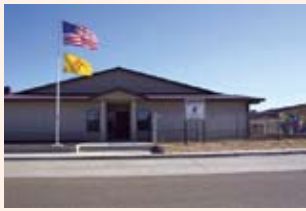
El Grito Head Start Building
