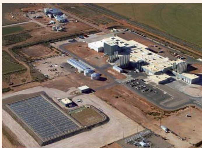
New Southwest Cheese Plant near Clovis. At $190 million, it is one of the largest dairy investments worldwide and the first of its kind that joined milk producers with cheese processors.
