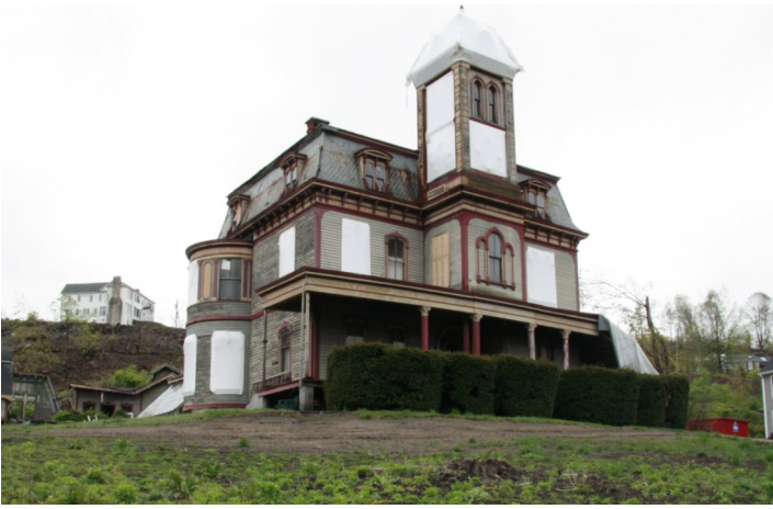
One of many historic buildings in Monson that had irreparable damage from the tornado. Zoning changes allowed Monson to rebuild to similar specifications. Credit: Larry Smith
