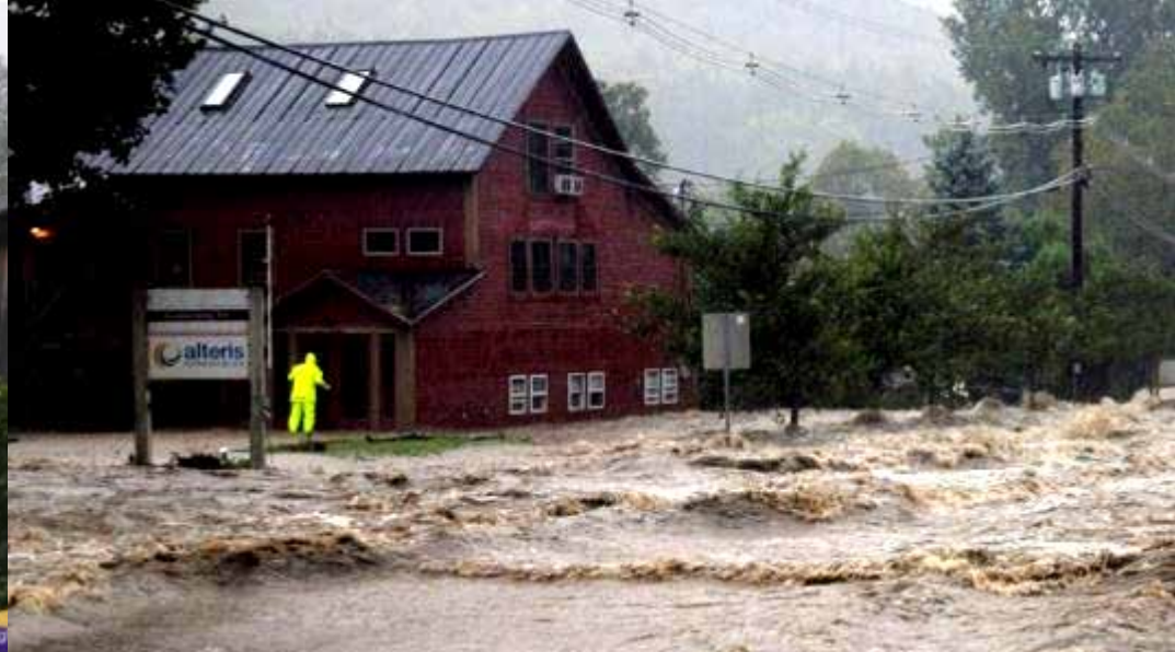
Green Hill, Tenn. Cata. & Brook Photo Studio Flooded. Photo: Jeff King
