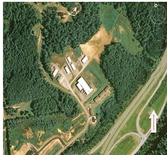
Park and Ride at I-79 and Sutton, West Virginia
