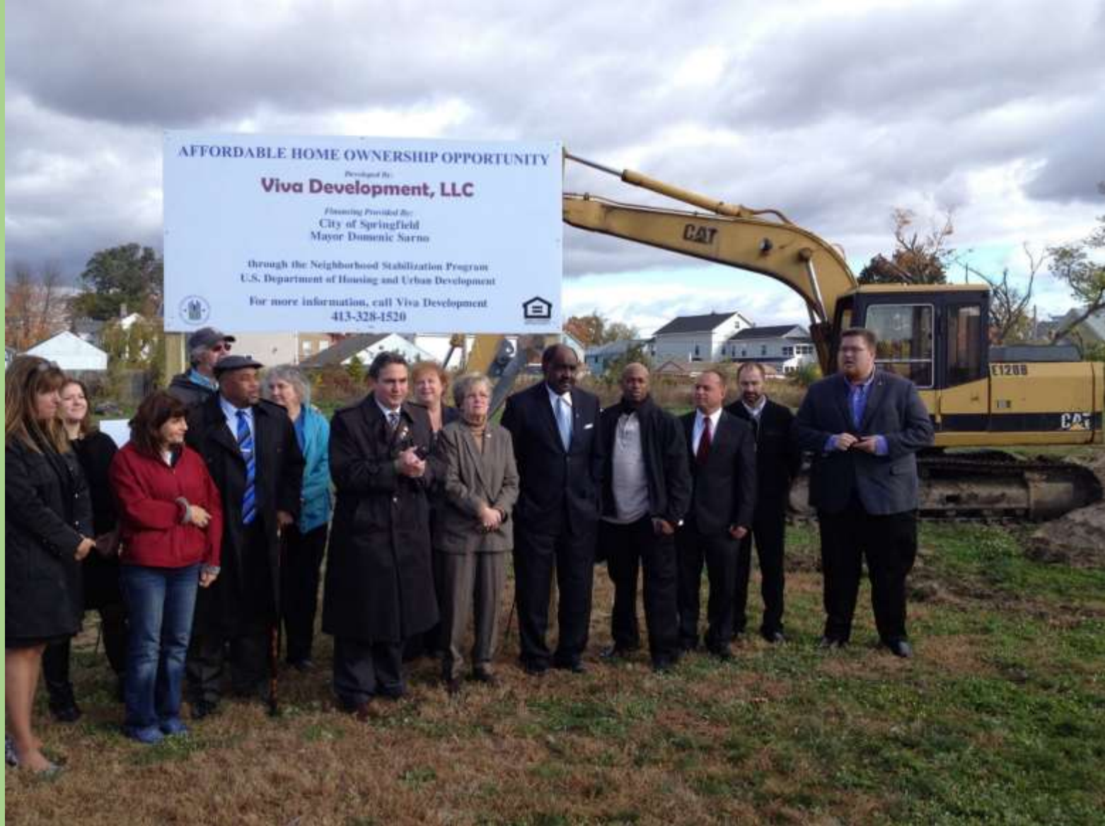
Groundbreaking for New Housing Funded through NSP and CDBG DR Funds
