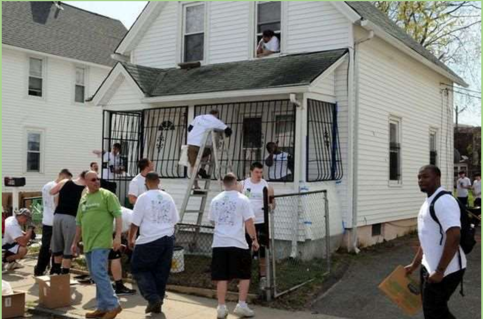
Partner with Nonprofit Partners & Volunteers Rebuild Together on Tyler Street
