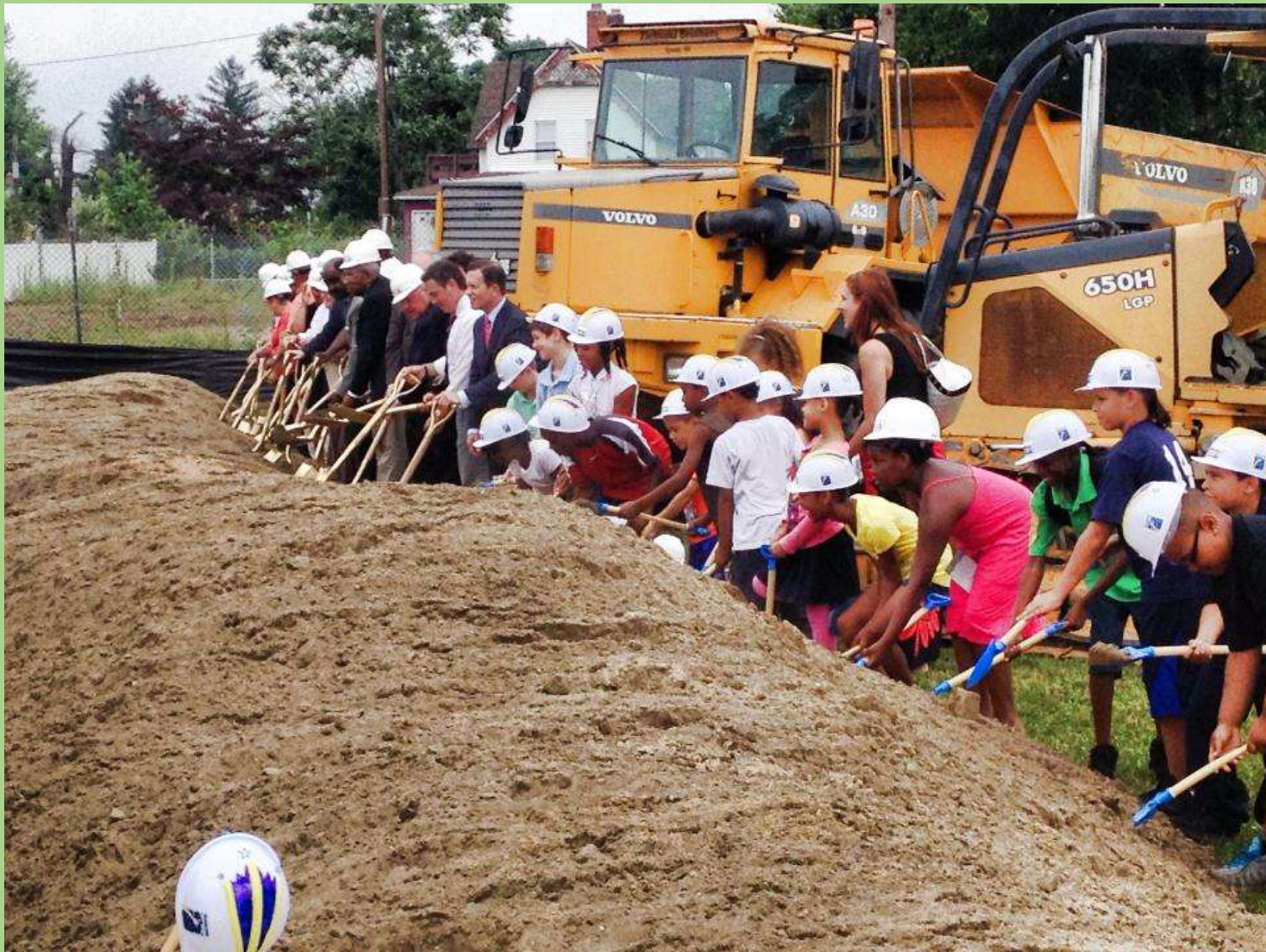
Groundbreaking for New School
