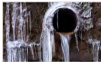
Preventing Frozen Pipes
