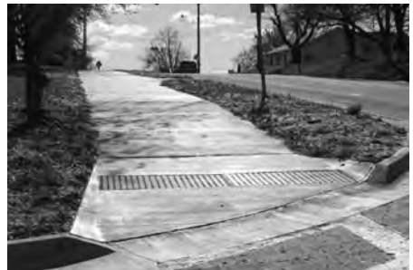
NW Missouri COG - Sidewalk Assessments, excellent condition
