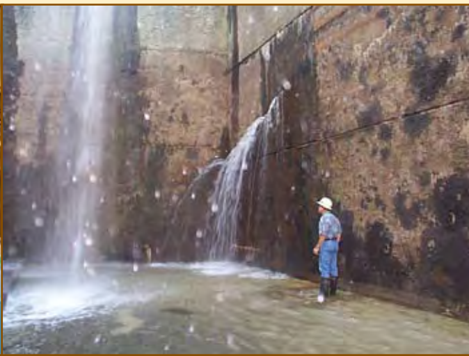
Left: The Army Corps of Engineers tests models of potential lock upgrade features. Right: An inspection shows some leakage at the current lock.
