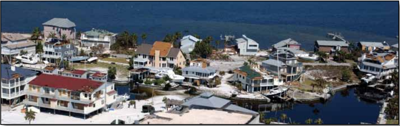
Pensacola, Florida, after Hurricane Ivan struck in 2004.
