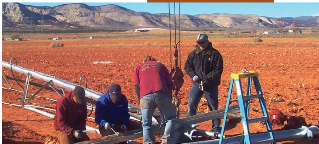
Workers assembling irrigation system
