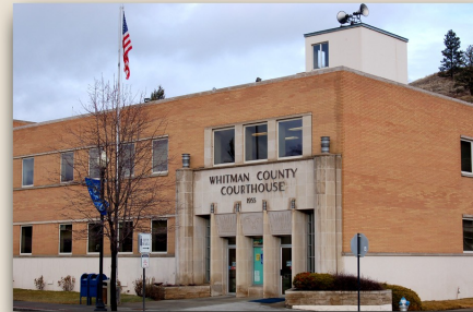
Whitman County Courthouse, Colfax
