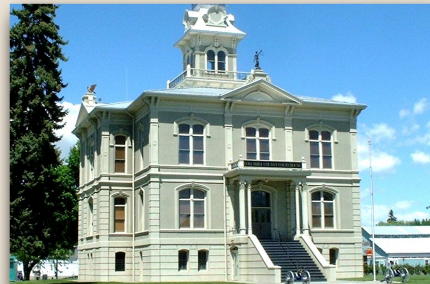
Columbia County Courthouse, Dayton
