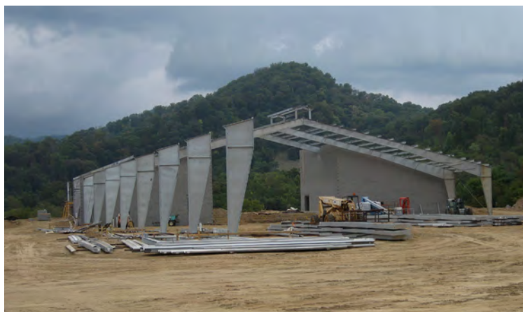
The WNC Regional Livestock Center under construction (photo courtesy of WNC Communities)
