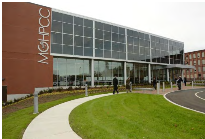
Massachusetts Green High Performance Computing Center, Holyoke Photo: MGHPCC
