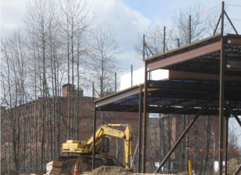
Construction of HealthSouth Rehabilitation Hospital at Ludlow Mills, Town of Ludlow Photo: Westmass Area Development Corporation
