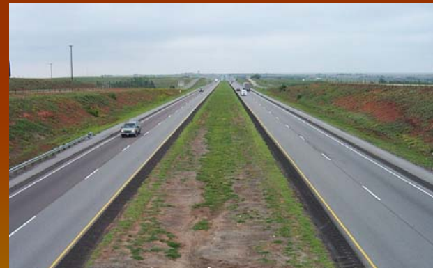
Lack of Development
